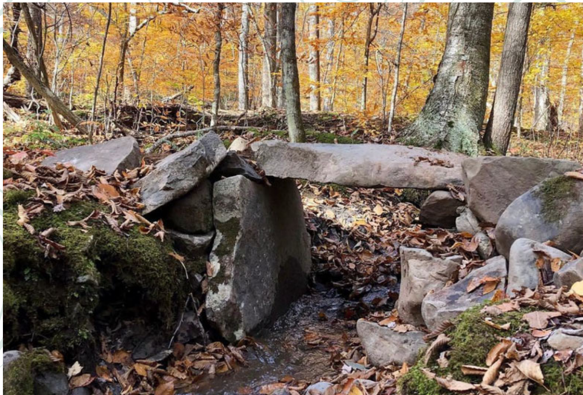
A photo of the largest bridge completed by the crew
