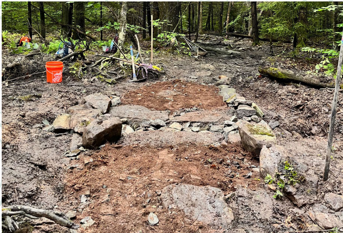
One of the newly completed drainage systems constructed by the crew
