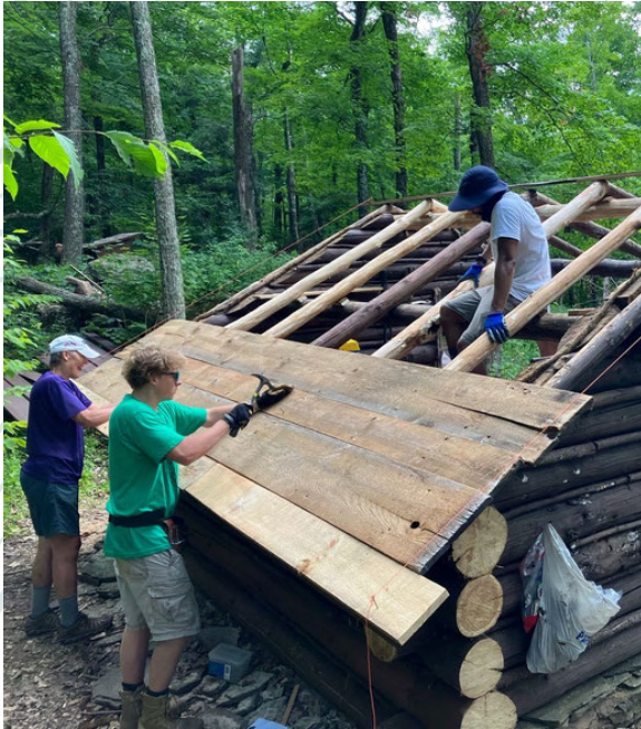
Liam nailing in the roof boards with volunteers
