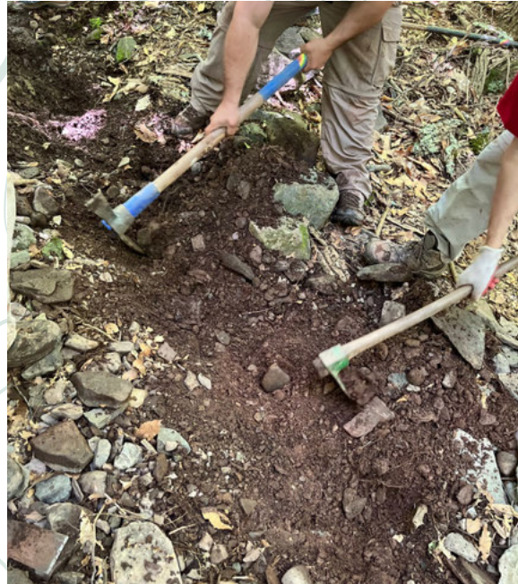
Digging another drainage path
