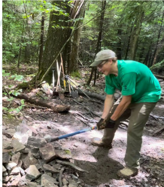
Liam making some crush for the treadway
