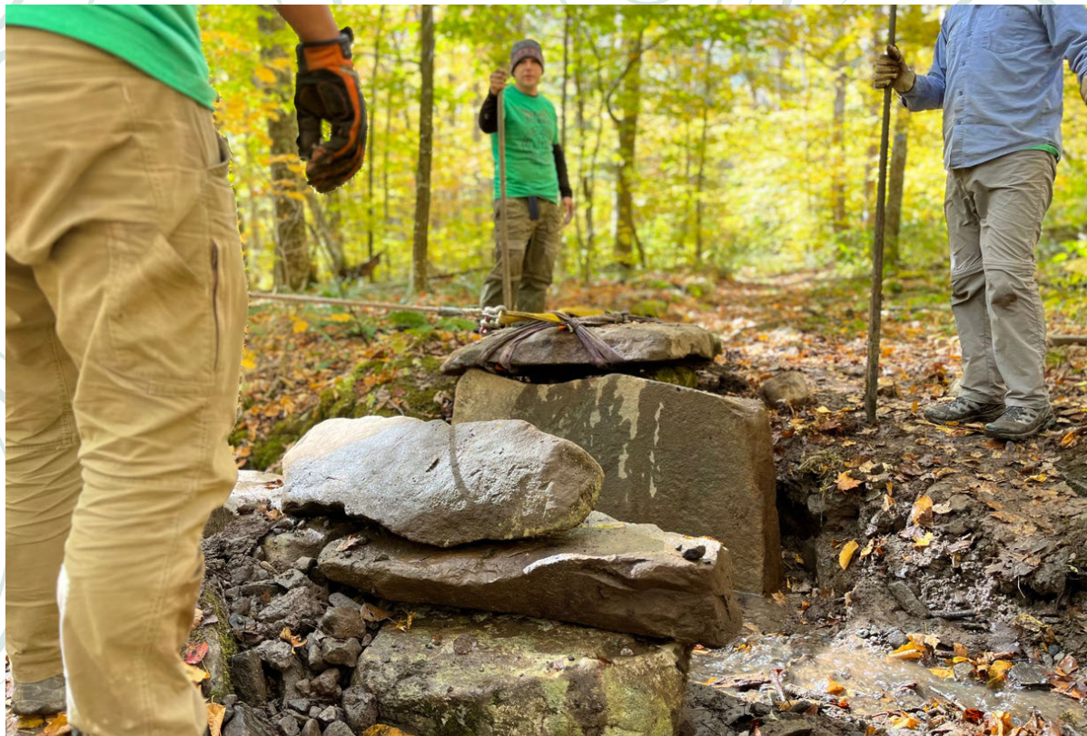
Josh, Brandon, and Andy determining the best route to guide the bridge rock to position it correctly
