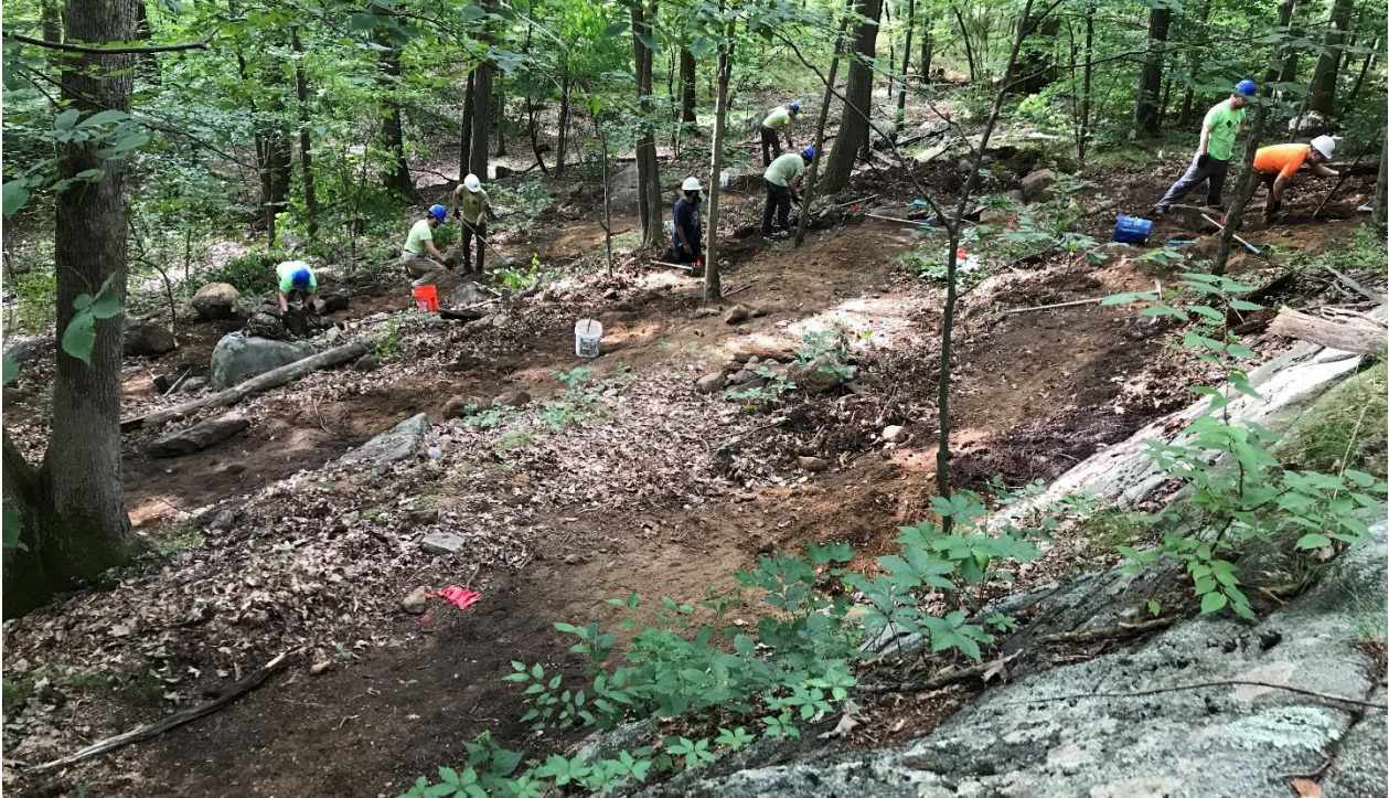
Stacked Climbing Turns Below Cliff
