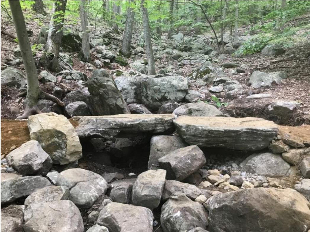
Stone Box Culvert
